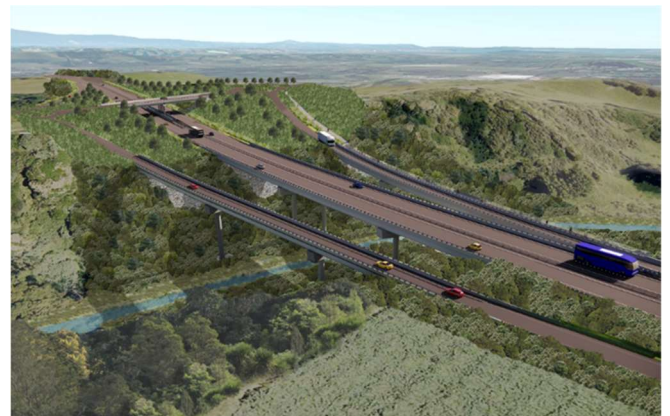
Artist impression - the overbridge interchange at Te Rangituanehu/ Minden Road is a collection of three bridges providing on and off ramps
